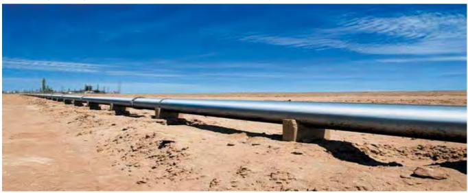
Korea EHT skin-effect trace heating is ideal for the freeze protection, temperature maintenance, and heat-up of materials transported by long-distance pipelines (25 km). Pipes can be above or below ground, submerged, and across all types of terrains. Applications Include the movement of materials in tank farms and storage terminals as well as piping between distant processing facilities in the chemical, petrochemical, oil, and natural/refined gas industries.
